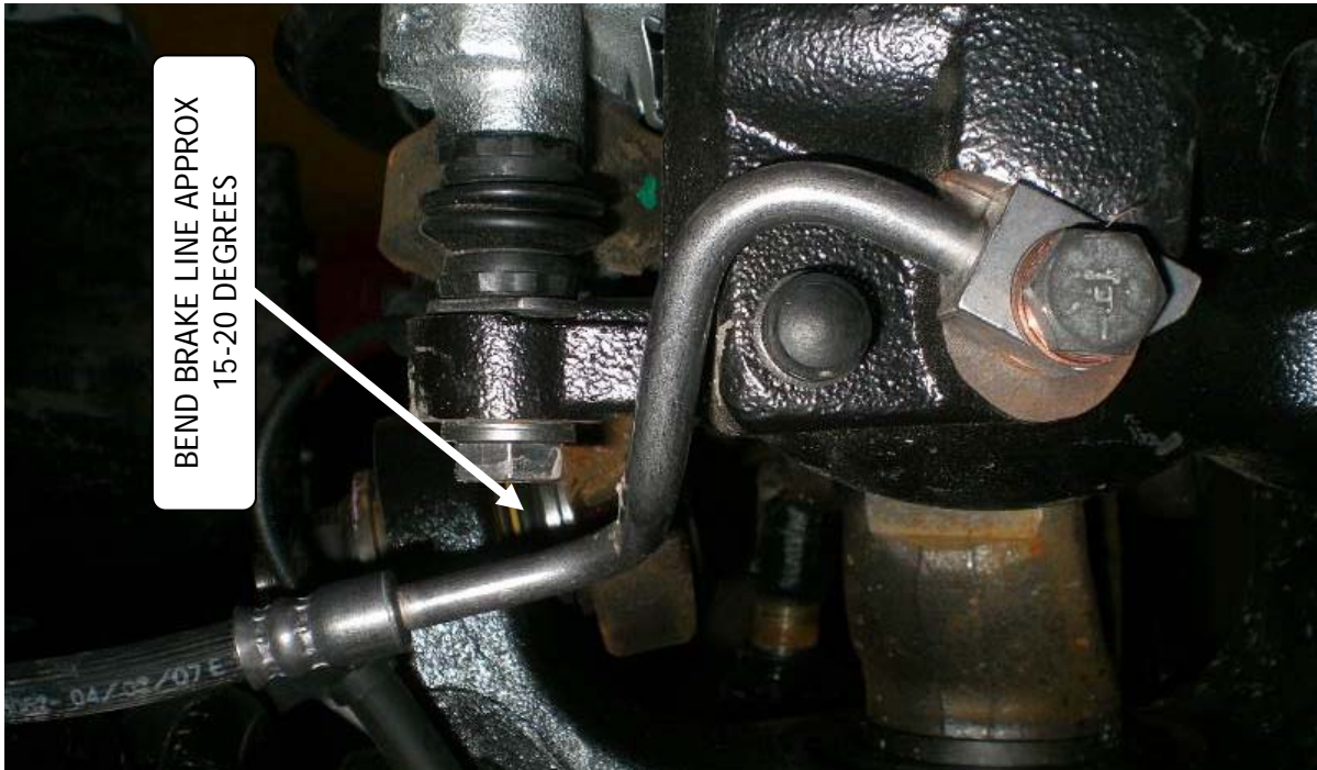
Figure 1 BRAKE LINE BENT AT APPROX. 15-20 DEGREES
